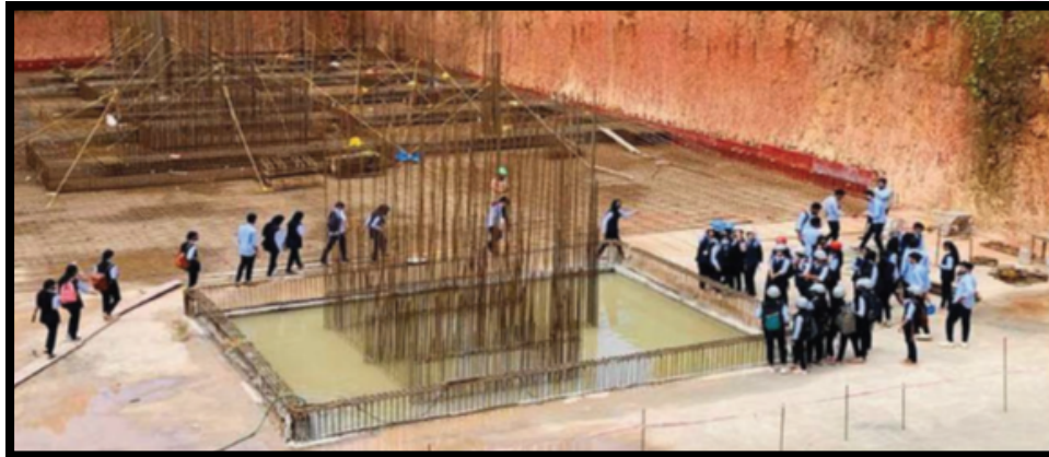
Site Visit- Kannur Municipal Corporation Building
